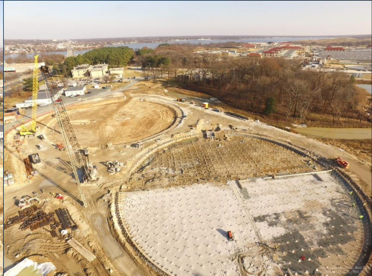
Tank 1 Stone Installation
