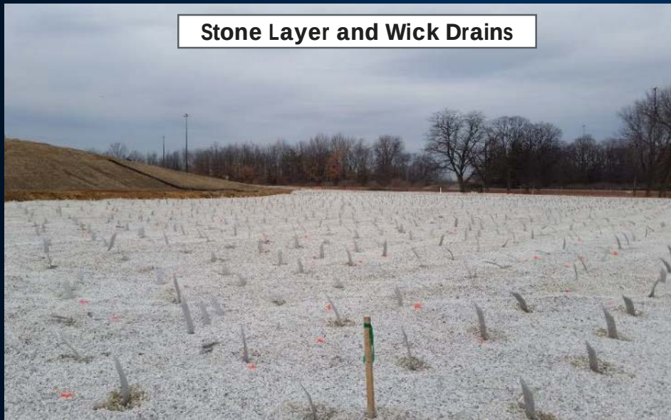
Wick Drain Installation
