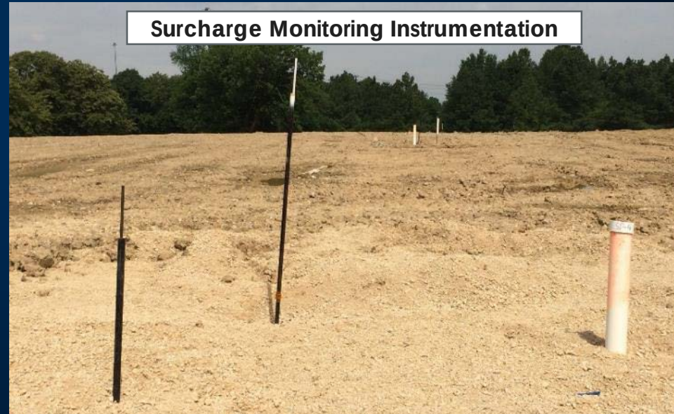
Surcharge Soil Placement
