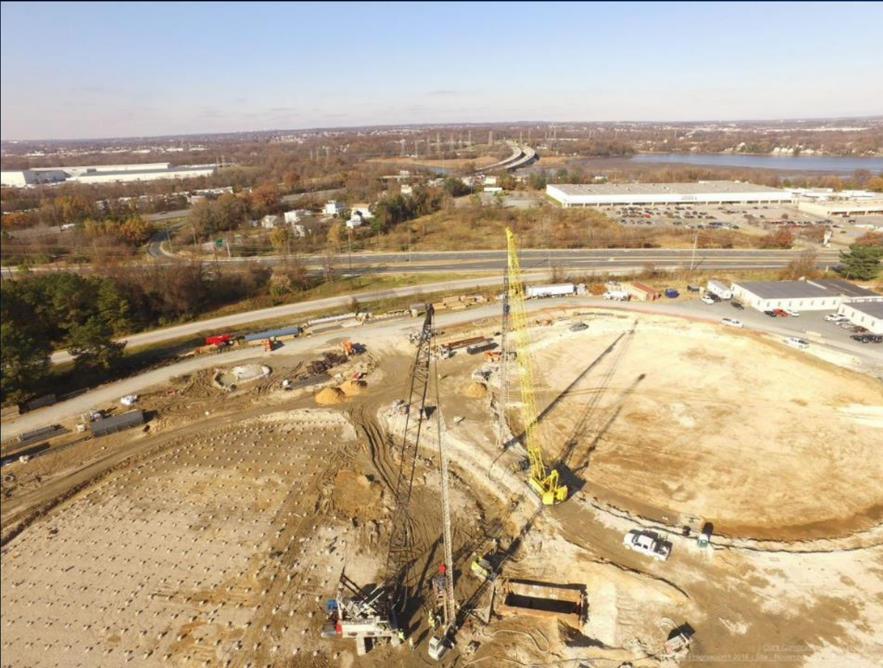
Tank 1 Pile Installation
