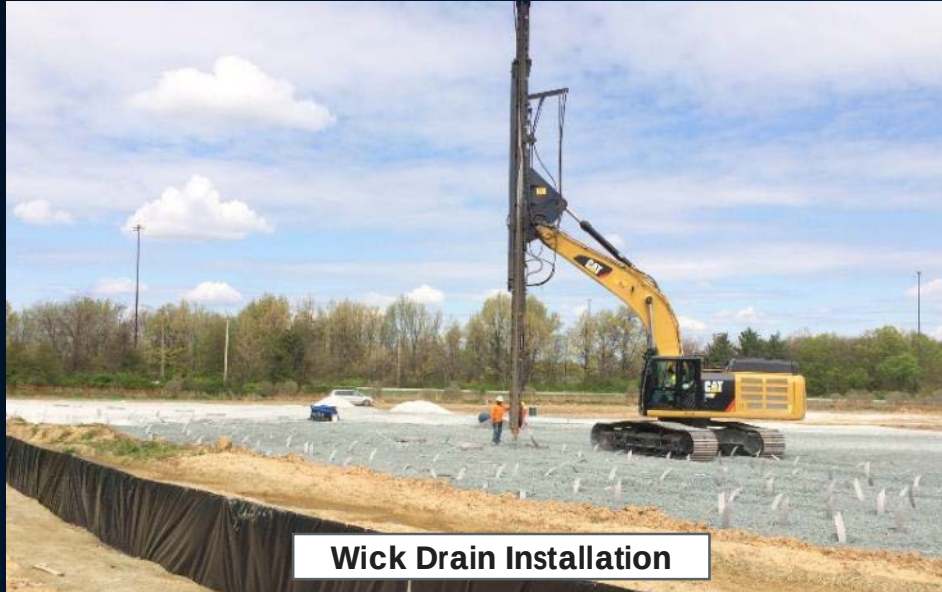
Stone Layer and Wick Drains
