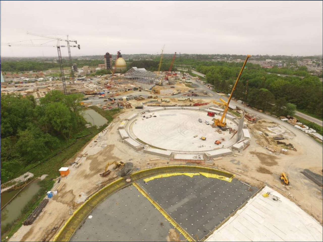
Tank 1 Slab Complete+Wall Panels – Tank 2 Slab
