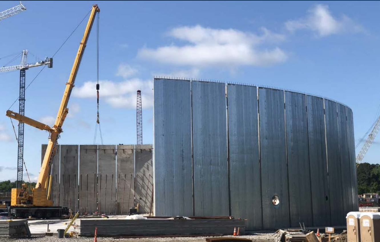
Tank 1 Wall Panel Erection
