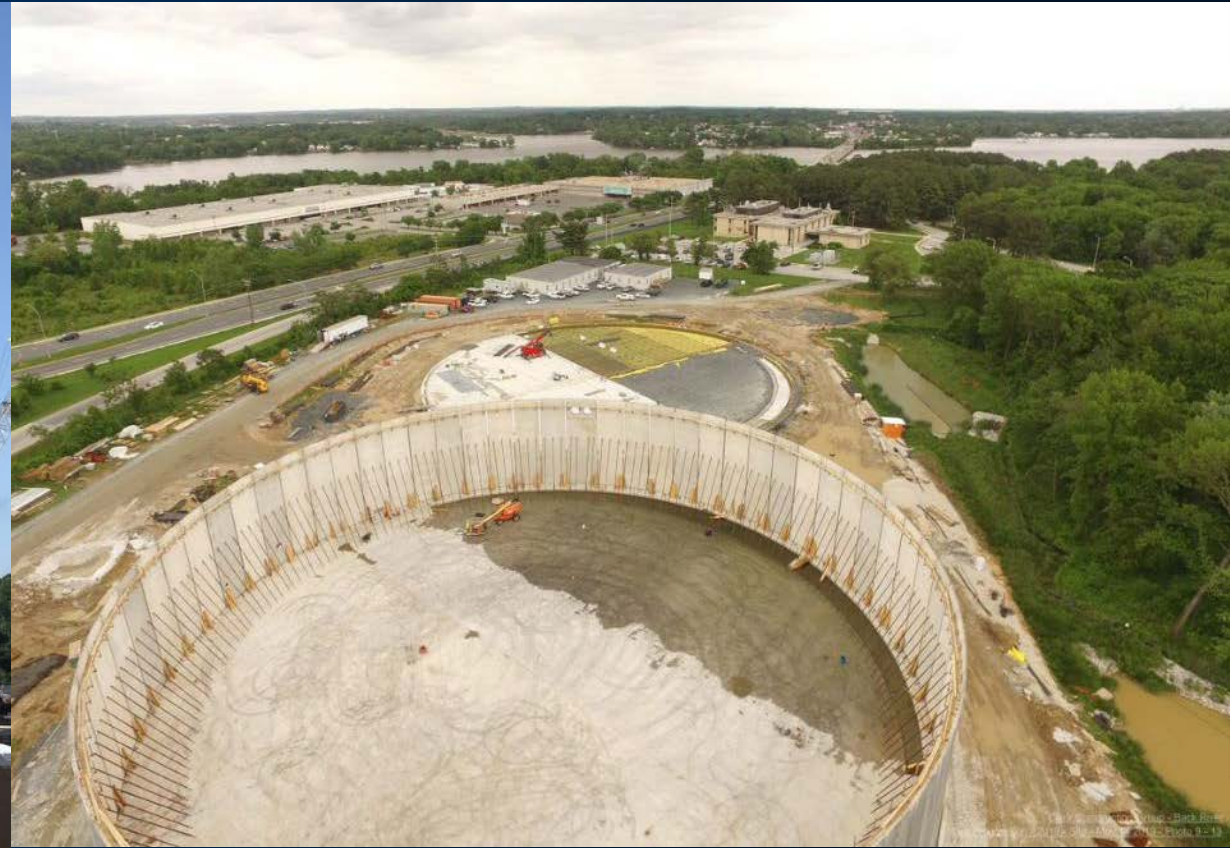
Tank 1 Wall Panels Up – Tank 2 Slab
