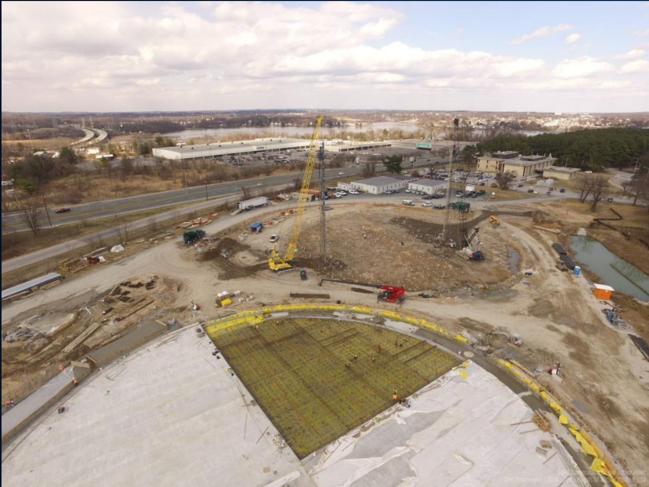
Tank 1 Slab Pours – Tank 2 Pile Install
